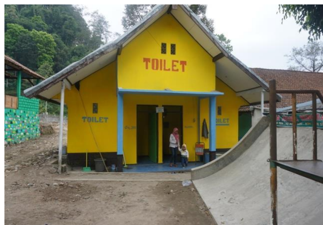
Gambar 6. Prasarana toilet umum
